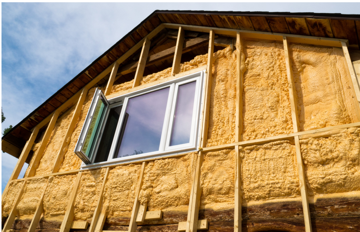
Spray foam insulation that conserves energy Photo Credit: PiLens Photo
